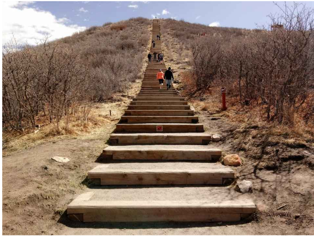
TIMBER STAIR RISERS WITH CRUSHED STONE
